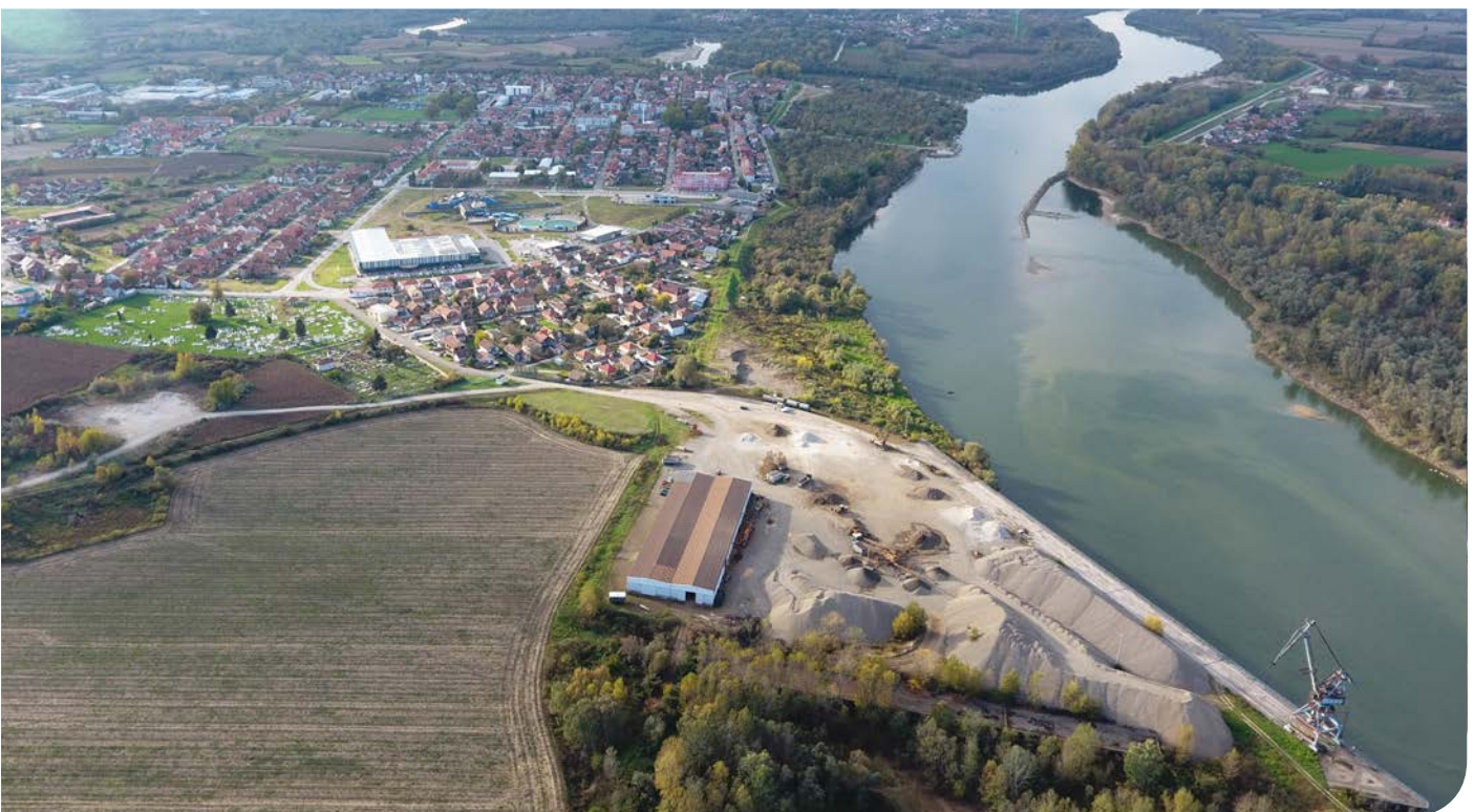
View on the Šamac Port
